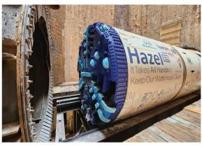
Hazel, the state-of-the-art tunnel boring machine, is currently constructing a 2-mile-long, 12-foot-wide tunnel to prevent combined sewage from polluting Alexandria's waterways.
