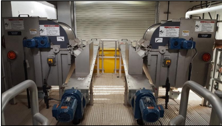
Figure 12-2 Scum Screen and Dewatering Press at the Cox Creek WRF, Anne Arundel County, MD
