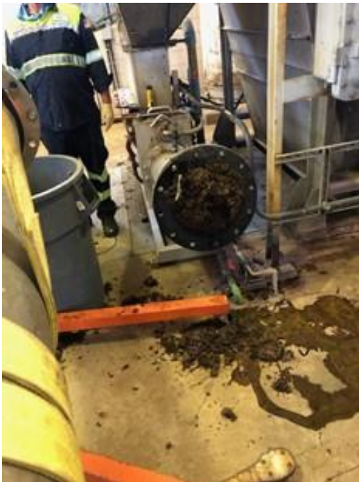
Figure 2-28 Clogging of Fine Screening System Due to Leaves During Peak Flow Conditions
