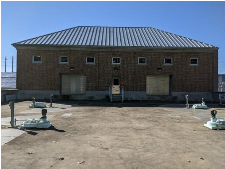
Figure 2-33 Building K Grit Deck
