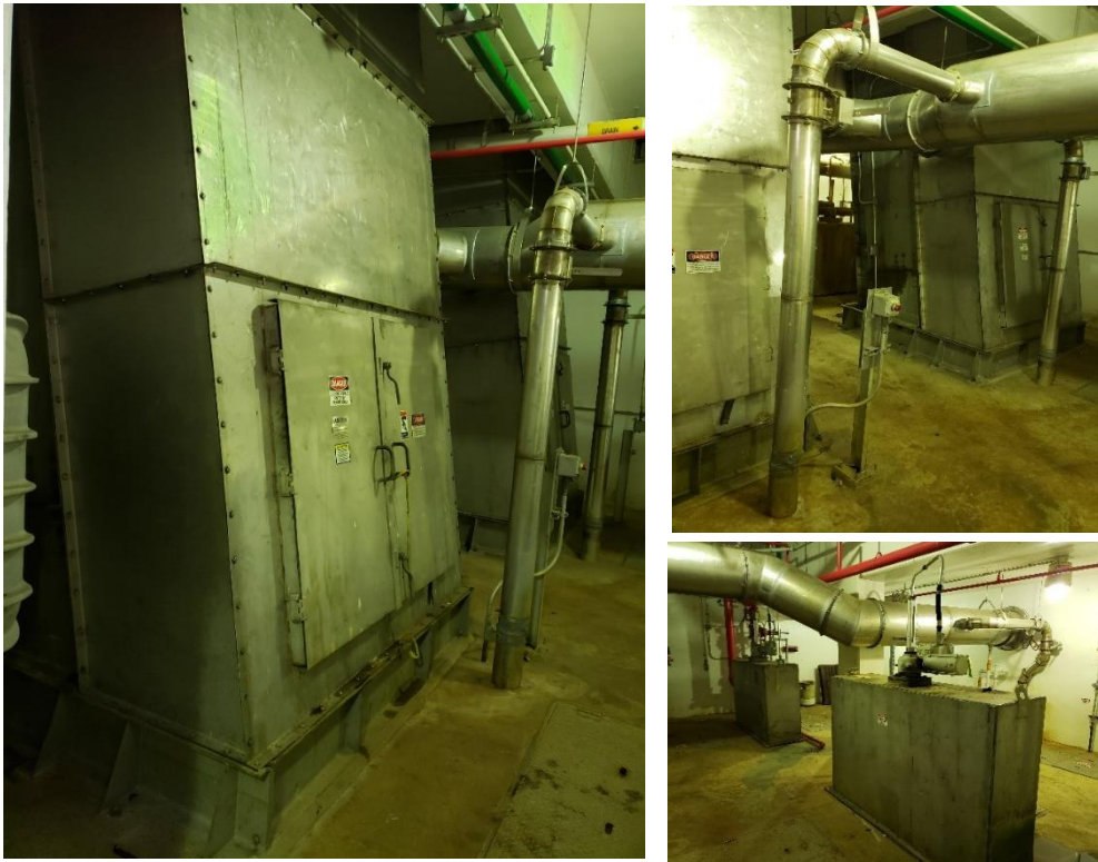
Figure 2-6 Existing Coarse Screening Area Basement
