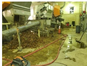
Figure 2-28 Clogging of Fine Screening System Due to Leaves During Peak Flow Conditions
