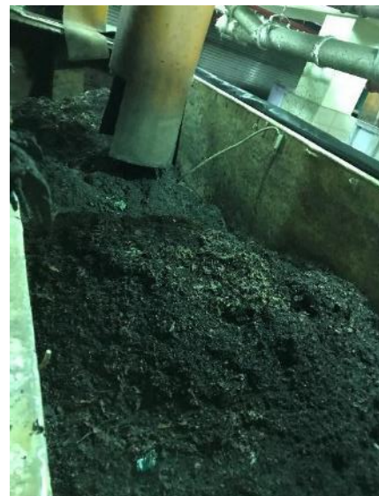
Figure 2-47 Screenings and Grit Piles
