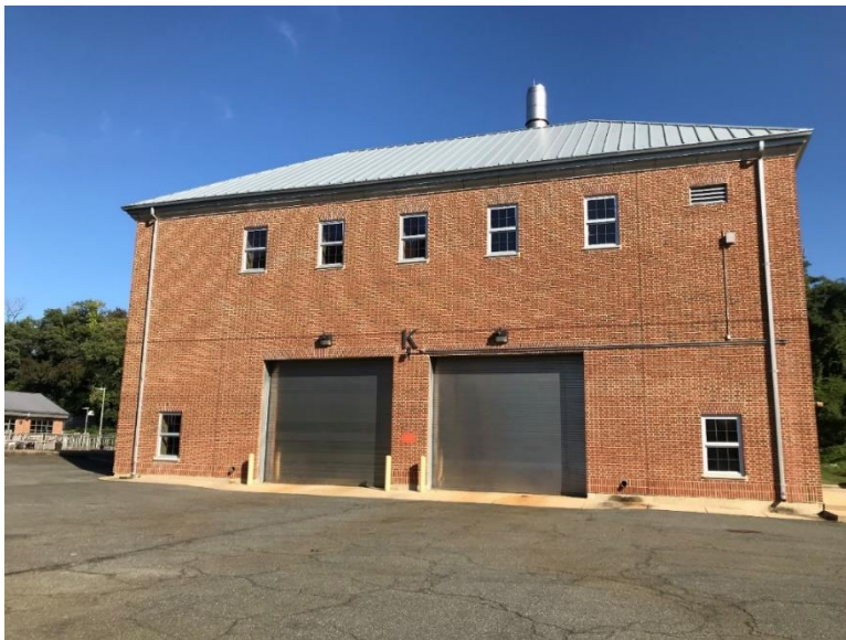
Figure 2-23 Existing Building K (Exterior View Looking North)
