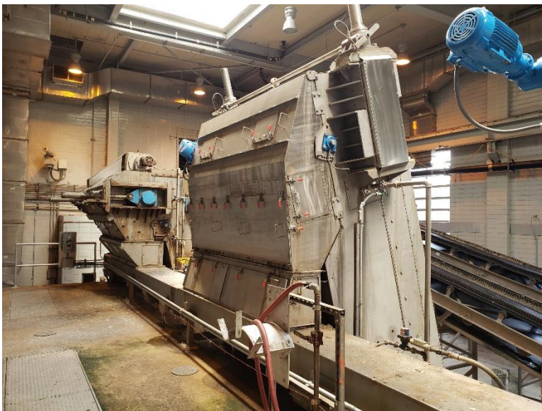
Figure 8-2 Existing (Left) and Renovated (Right) Mechanical Screens at DC Water
