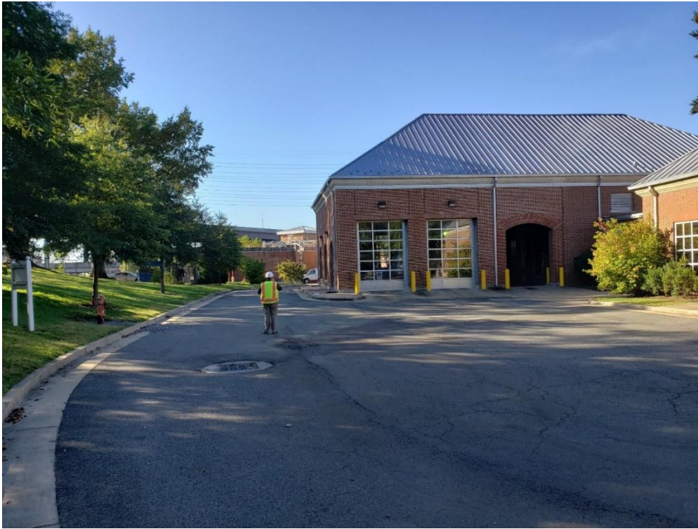
Figure 2-4 Existing Coarse Screen Room (Exterior View Looking South)
