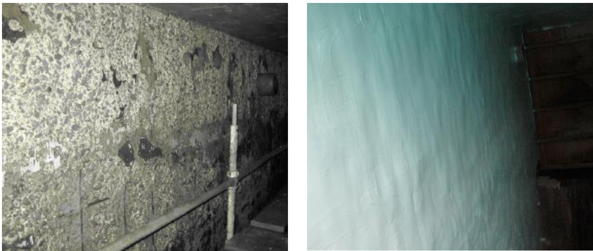
Figure 7-2 Quadex Structure Guard® Before and After Photos
