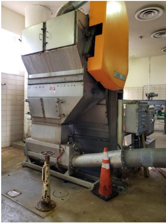
Figure 2-24 Existing Fine Screens with Washer/Compactors
