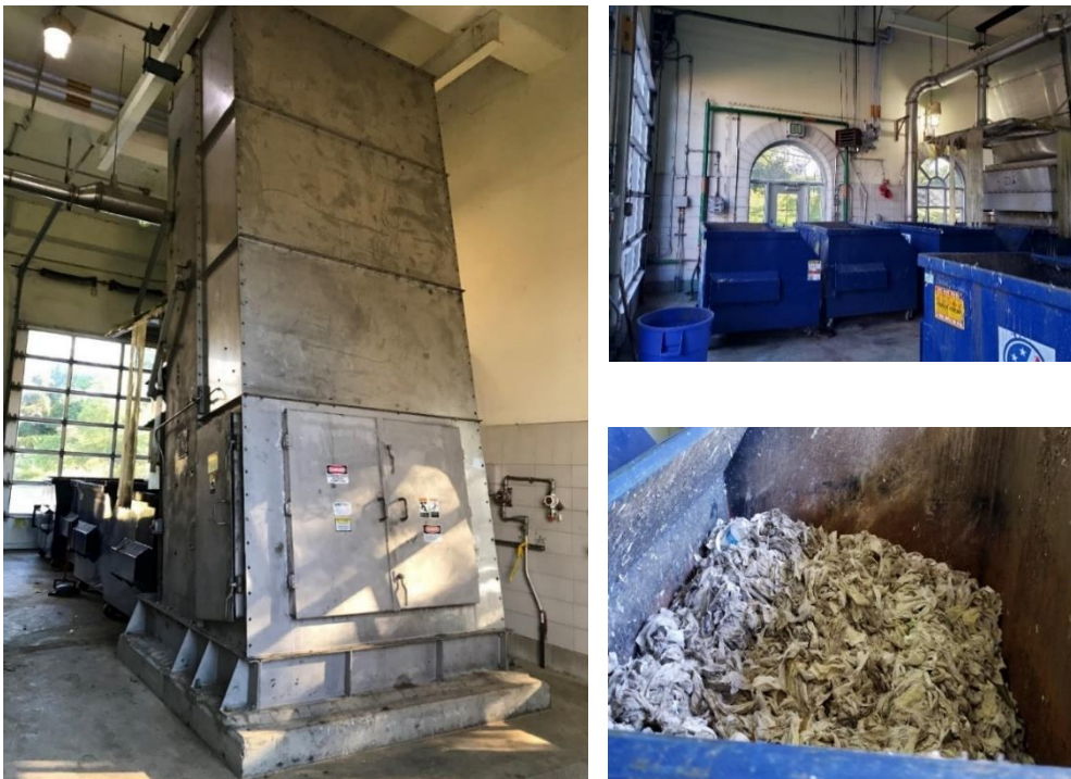
Figure 2-5 Existing First Floor Coarse Screen Room
