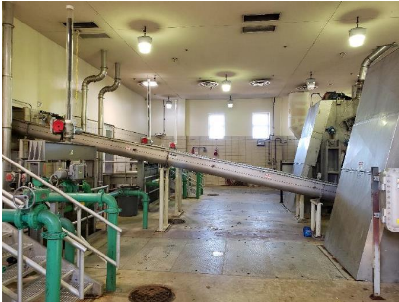
Figure 2-44 Fine Screens Screening Conveyors from the Screening Room to the Cyclone Classifier Room
