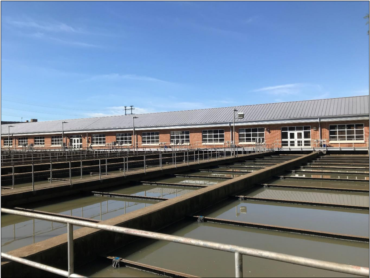
Figure 2-50 Primary Settling Tanks and Primary Weir Observation House
