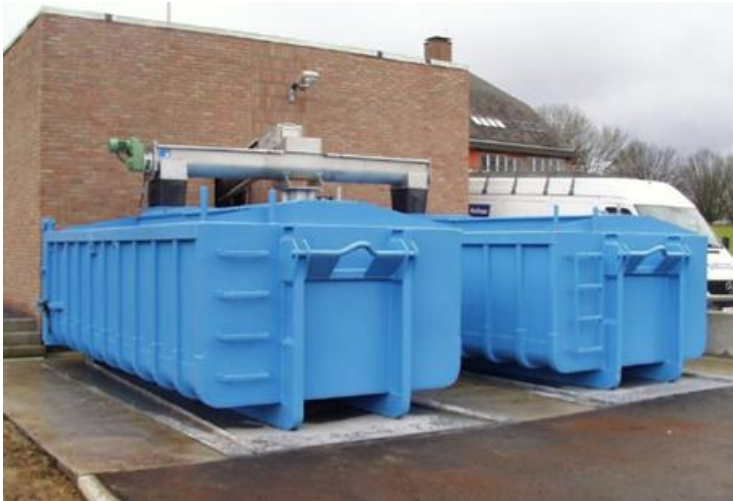
Figure 10-2 Self-Leveling Roll-Off Container Installation (Courtesy Schwing Bioset)
