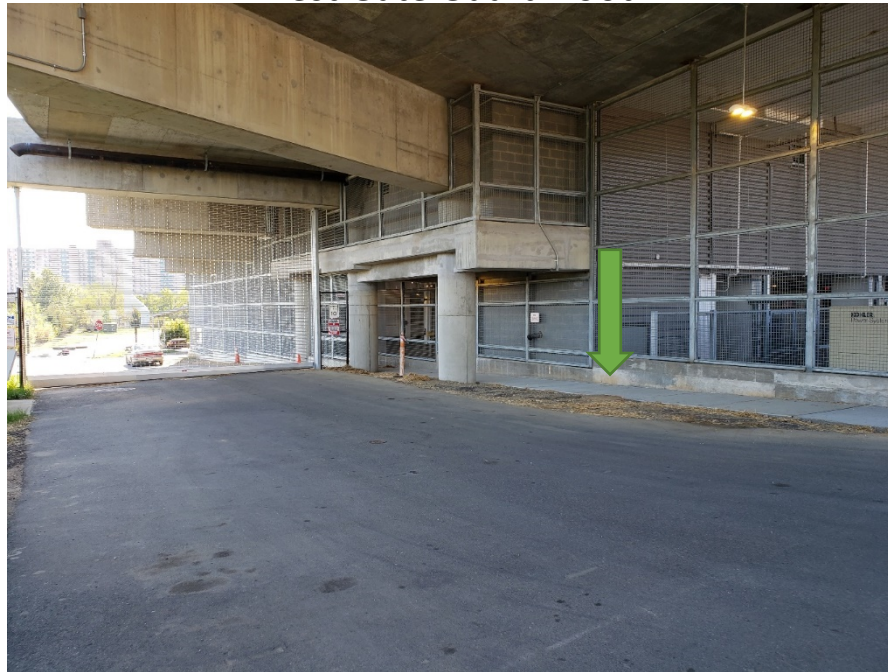
West Gate Guard Booth
