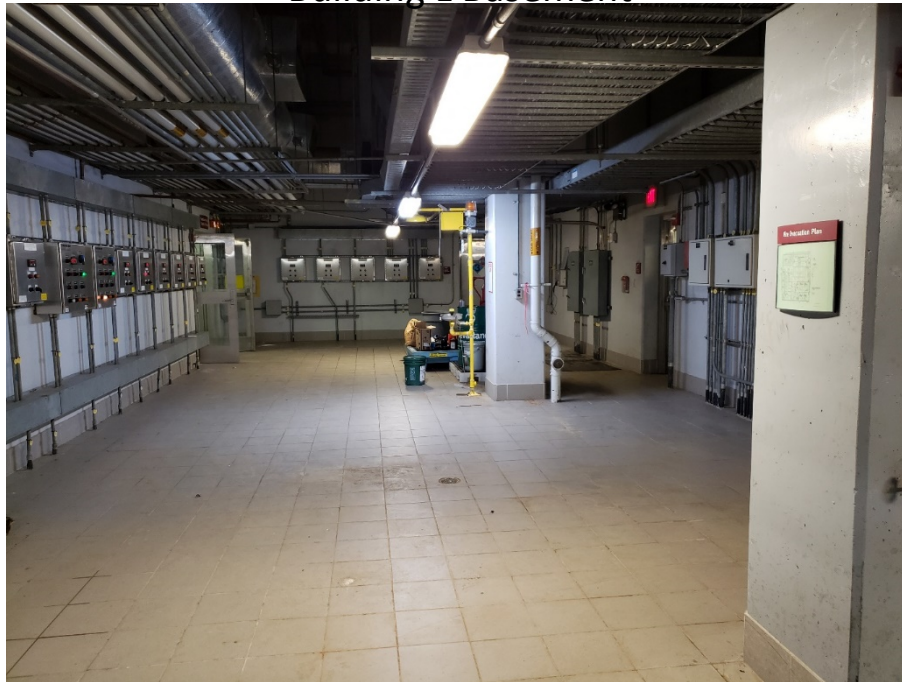
Building L Basement
