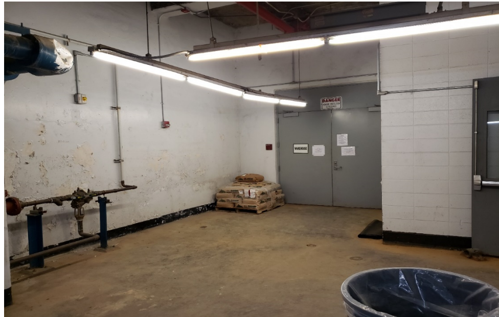
NEW Shelter Point Building G Basement
