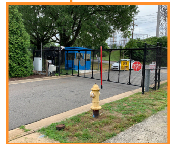
WRRF Site Security and Access Project New gates and guard booths installed and operational in September 2020
