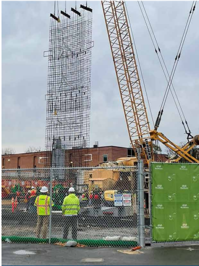
Reinforcing Cage
