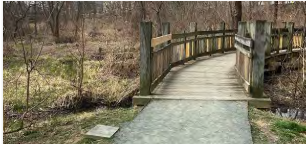
Photo 3. End of Asphalt Path Along Hooffs Run
