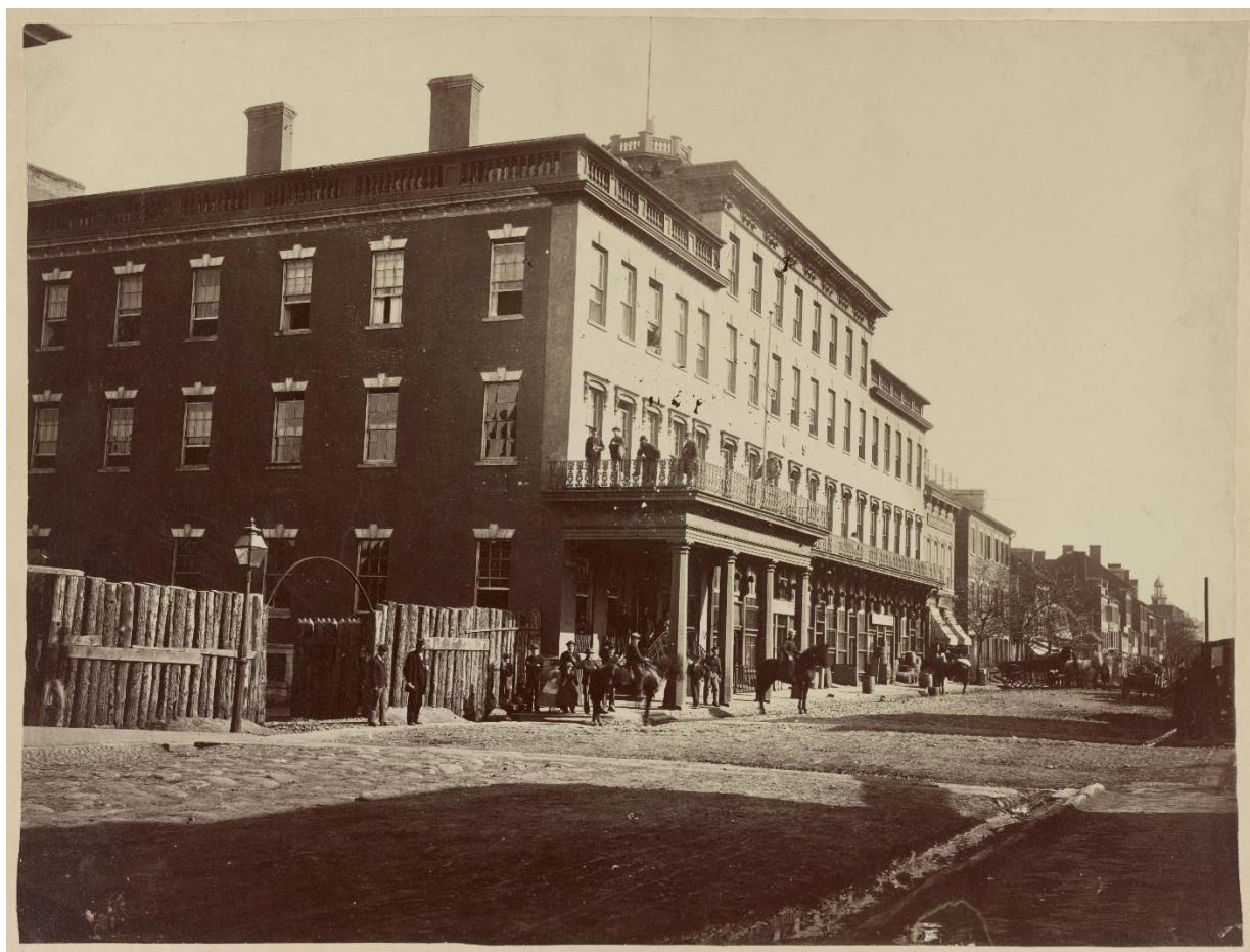
Figure 1 - Mansion House, Alexandria, Va. during the Civil War. Note the gutter at the bottom-right of the image that passes under the side street. (Library of Congress Prints and Photographs Division)
