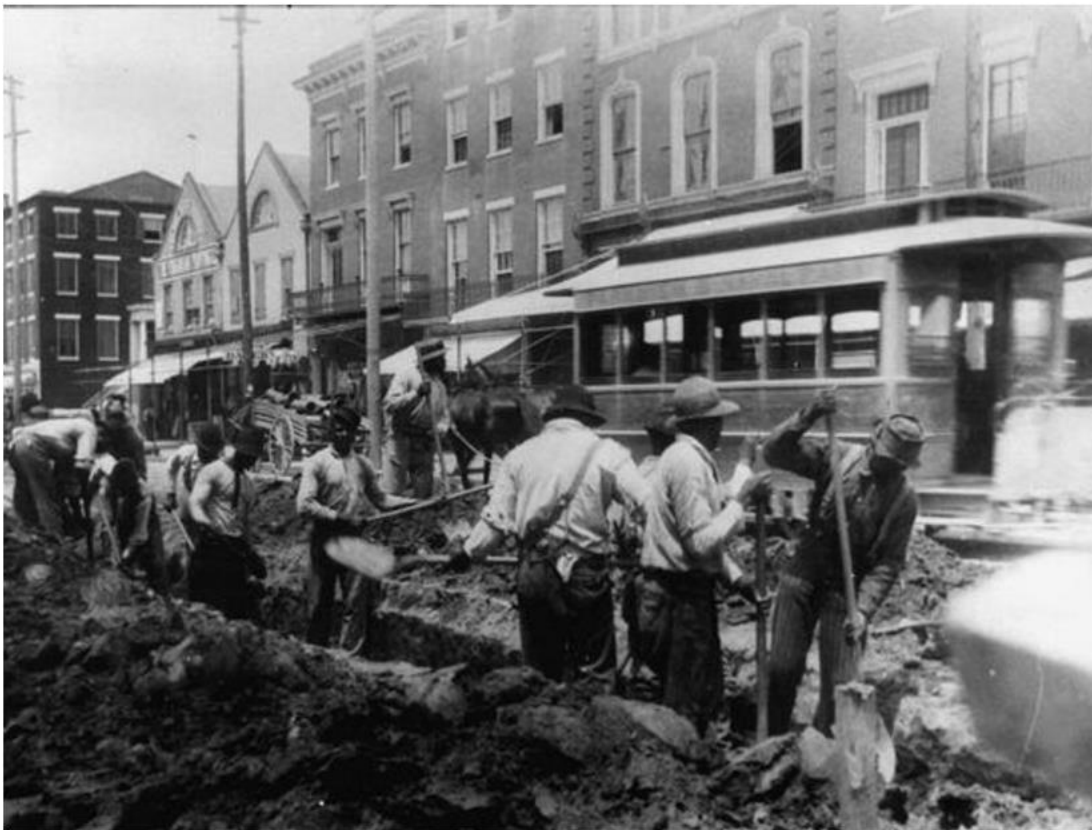
Figure 2 - Laying Sewer Main in Portsmouth, Virginia. Alexandria's sewer mains were constructed using open ditch techniques as is seen here in Portsmouth, Virginia. (Library of Virginia)
